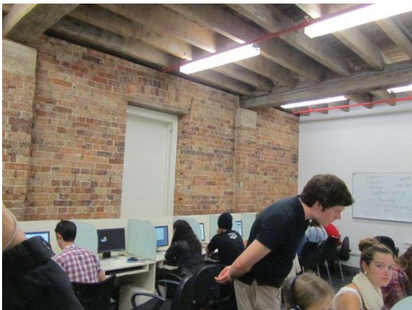
ONE OF THE SOUTHERN CLASSROOMS SHOWING THE REAR WALL WITH BRICK AND SANDSTONE PIERS AND INFILLED FORMER WINDOW. TIMBER FLOORBOARDS, BEAMS AND JOISTS ARE EXPOSED ABOVE.
