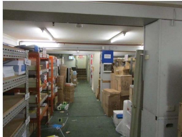
BASEMENT VIEW WEST TO THE FIRE STAIR.
