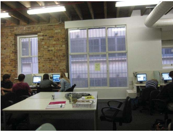
INTERIOR WESTERN ELEVATION SHOWING THE FACEBRICK AND PART RENDERED FINISH AND ALTERED CASEMENT WINDOWS (SOUTHERN STORE)
