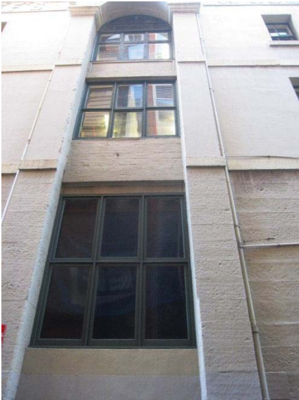
THE MODIFIED CENTRAL LOADING BAY
