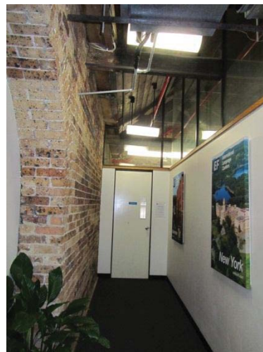
VIEW WEST SHOWING CONTEMPORARY PARTITIONING AND SIGNIFICANT ROOF SYSTEM
