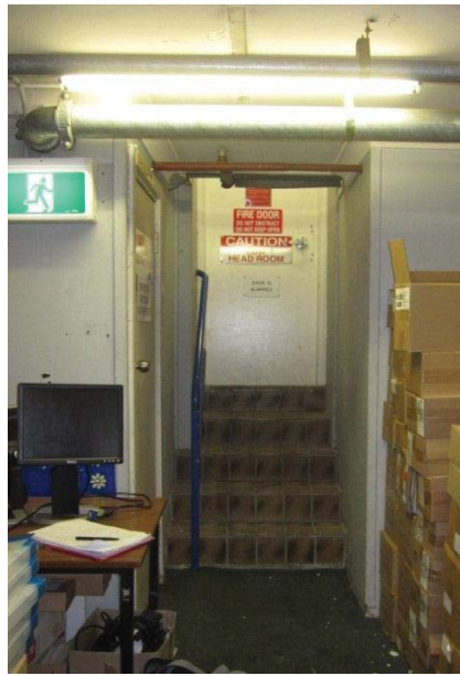
THE FIRE STAIR (TO LOFTUS LANE) AND SPRINKLER CONTROL ROOM AT LEFT.
