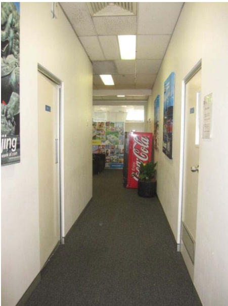
VIEW EAST ALONG THE HALL TO CLASSROOMS (AT RIGHT) AND WCs (AT LEFT) (SOUTHERN STORE) SHOWING CONTEMPORARY FIT OUT AND FINISHES
