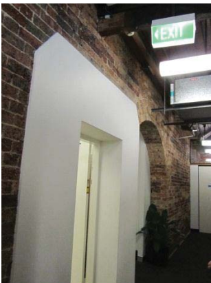
VIEW OF THE CENTRAL ARCH AND NEW OPENING TO THE STAIR HALL
