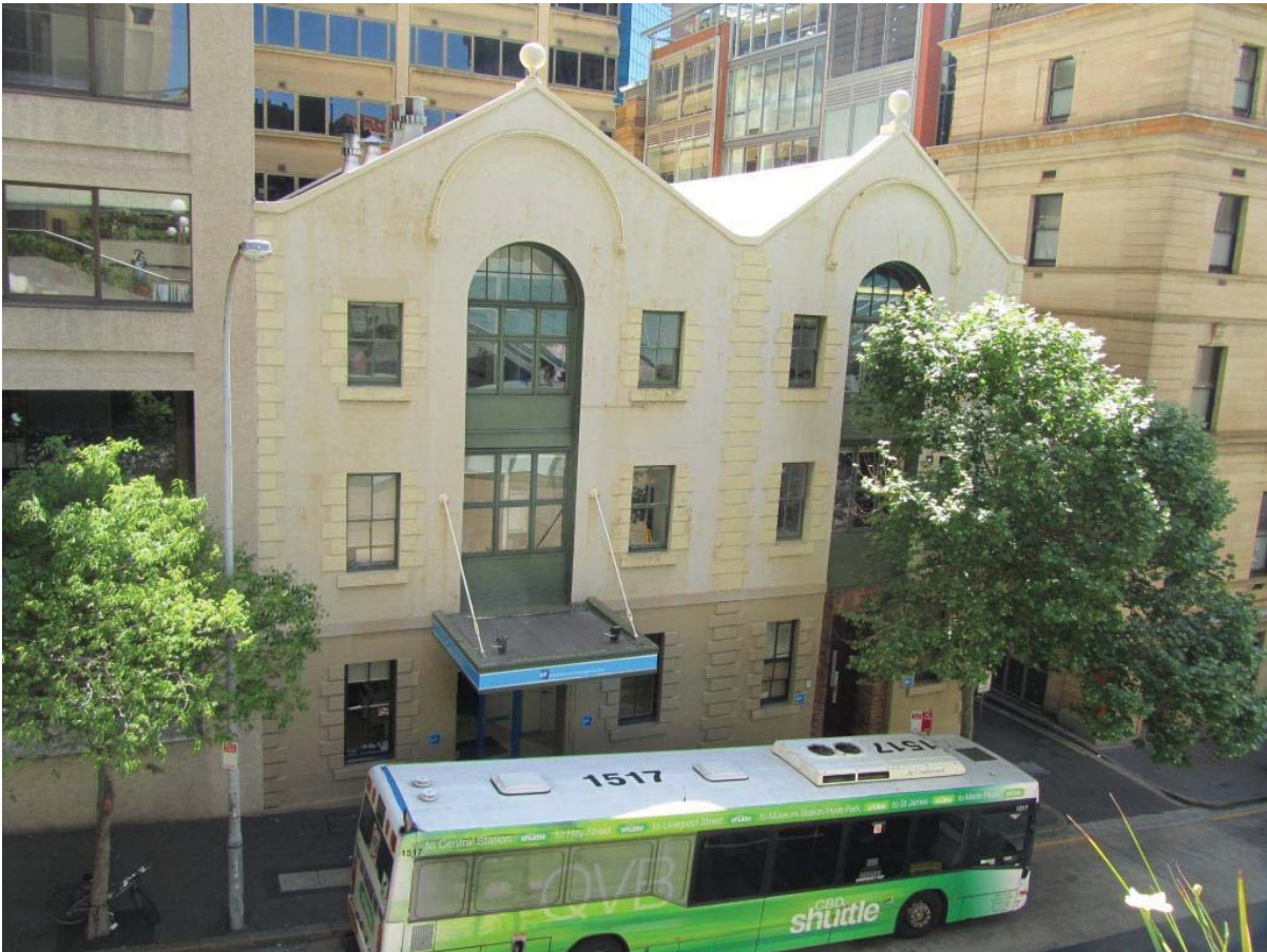
THE PRINCIPAL/ EASTERN ELEVATION
