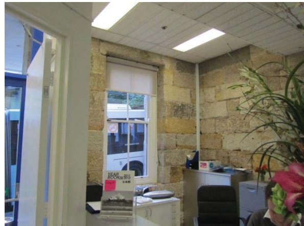
THE GROUND FLOOR OFFICE AREA, SHOWING THE ENTRY, SANDSTONE WALLING AND TIMBER DOUBLE HUNG WINDOW (TO EAST ELEVATION)
