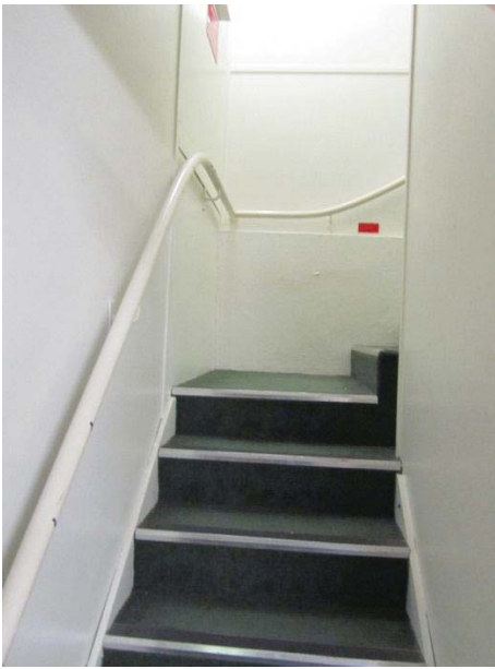
BASEMEN STAIR TO THE GROUND FLOOR
