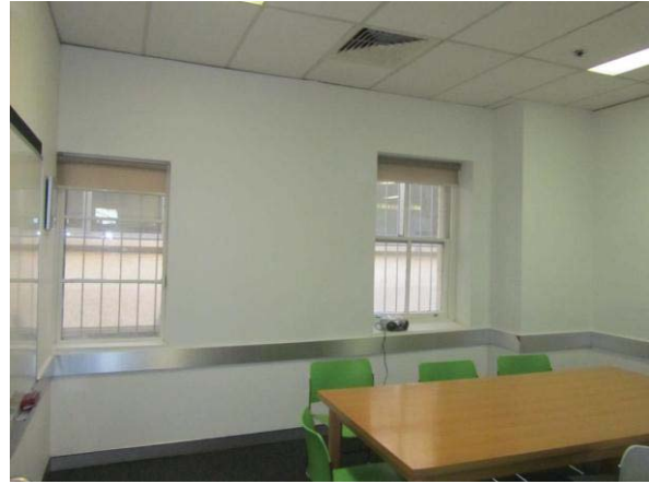
CLASSROOM AT THE WESTERN END OF THE SOUTHERN STORE. THE CENTRAL ARCHED WINDOW/ FORMER LOADING BAY HAS BEEN PARTIALLY INFILLED AND REPLACED WITH A SMALLER WINDOW (LEFT), AND BISECTED BY THE CLASSROOM PARTITIONING
