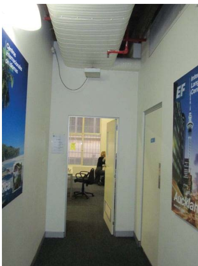
VIEW WEST IN THE SOUTHERN STORE SHOWING CONTEMPORARY PARTITIONING AND SERVICES
