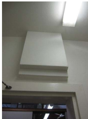
DETAIL OF THE CUT BRICK PIER ABOVE THE NEW OPENING TO THE STAIR HALL.
