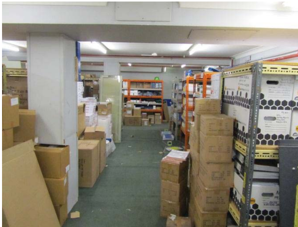
BASEMENT VIEW EAST. THE ORIGINAL HARDWOOD TIMBER COLUMNS ARE ENCASED WITHIN PLYWOOD CLADDING
