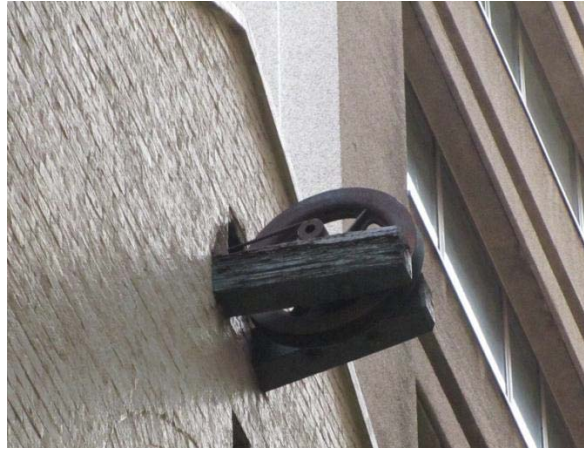
DETAIL OF THE RETAINED CATHEAD PULLEY ON THE SOUTHERN STORE
